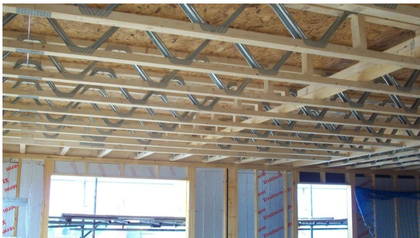
Fig. 14 – Metal web joists
